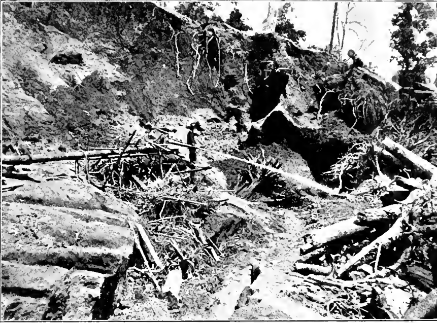
Fig. 2.—TWO-INCH MONITOR AT WORK. (Note depth of soil).
